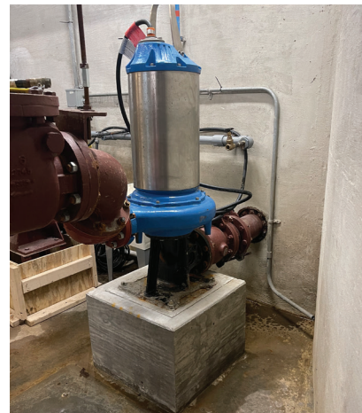
After installation of envie 3 pump
