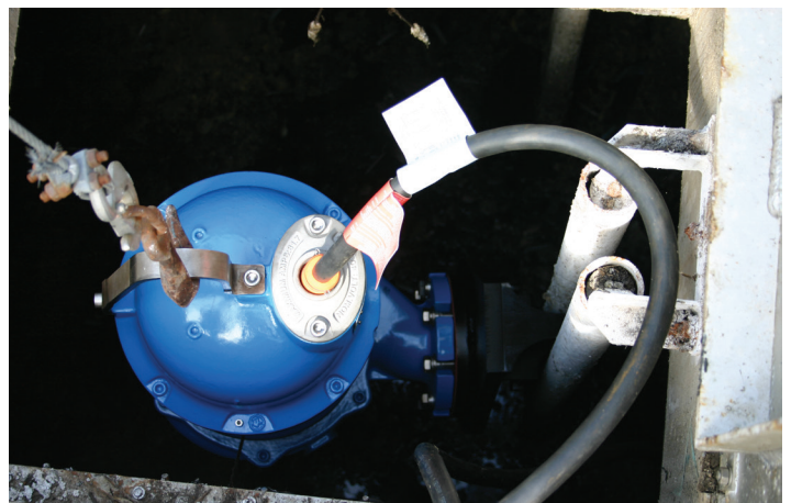
SITHE chopper pump being lowered into it's stations
